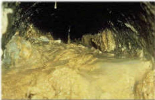
The same thing can happen to the City of Camarillo wastewater collection system. Most blockages in the wastewater system can be traced back to FOG. The result can have damaging effects throughout the system creating sewage spills, manhole overflows or backups into homes or businesses. Too much grease and oil can also create the need for increased maintenance of the sanitary sewer lines, increasing costs to all customers
